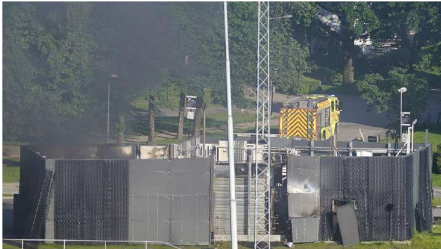
Fig.37.: The pressure wave lifted up the roof of the compartment and through away in several hundred meters [photo: Heiko Junge / NTB scanpix]
